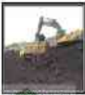
Grade 4-5 Digging, Trenching, and Earth Retention
